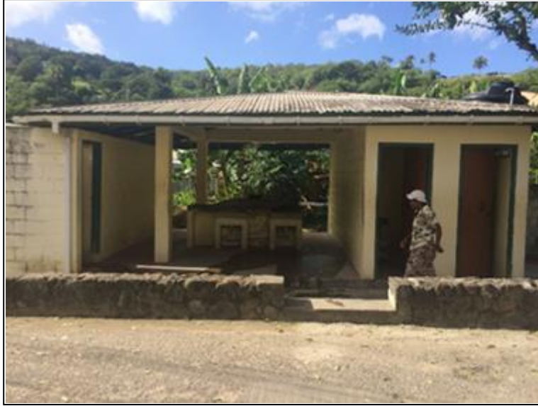
Figure 8: Washroom #2 is on the outskirts of the commonly flooded area
