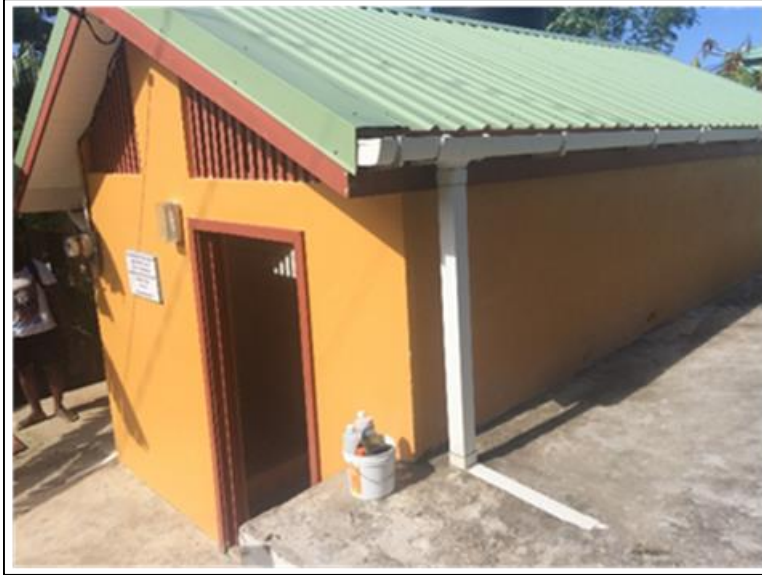
Figure 10: Washroom #3 is on higher ground and not in danger of flooding
