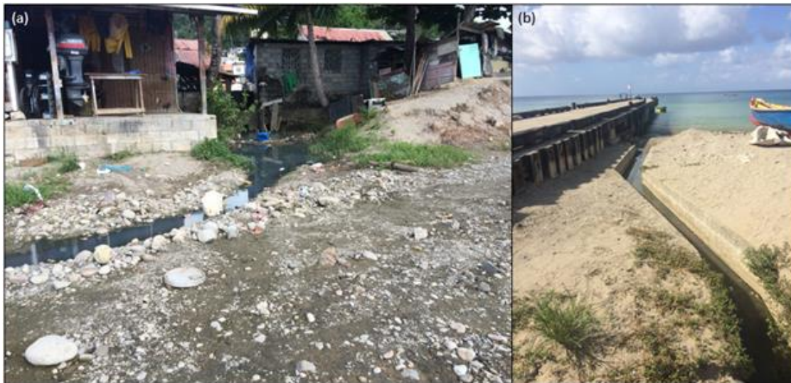
Figure 5: Stormwater, greywater and wastewater draining to river (a) and ocean (b) via street stormwater drains
