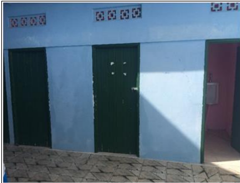
Figure 11: The old church is located with in the common flood area. It has no visible riser and has never been pumped before. The effluent appears to discharge into the open gutters.
