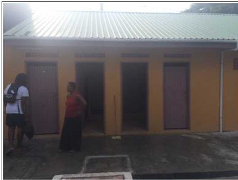
Figure 7: Washroom #1 is on the oceanfront and is commonly flooded
